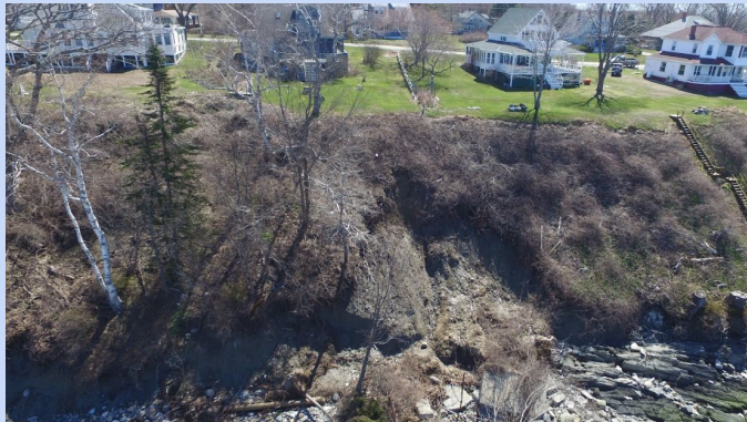
Bluff erosion; view from front beach.
